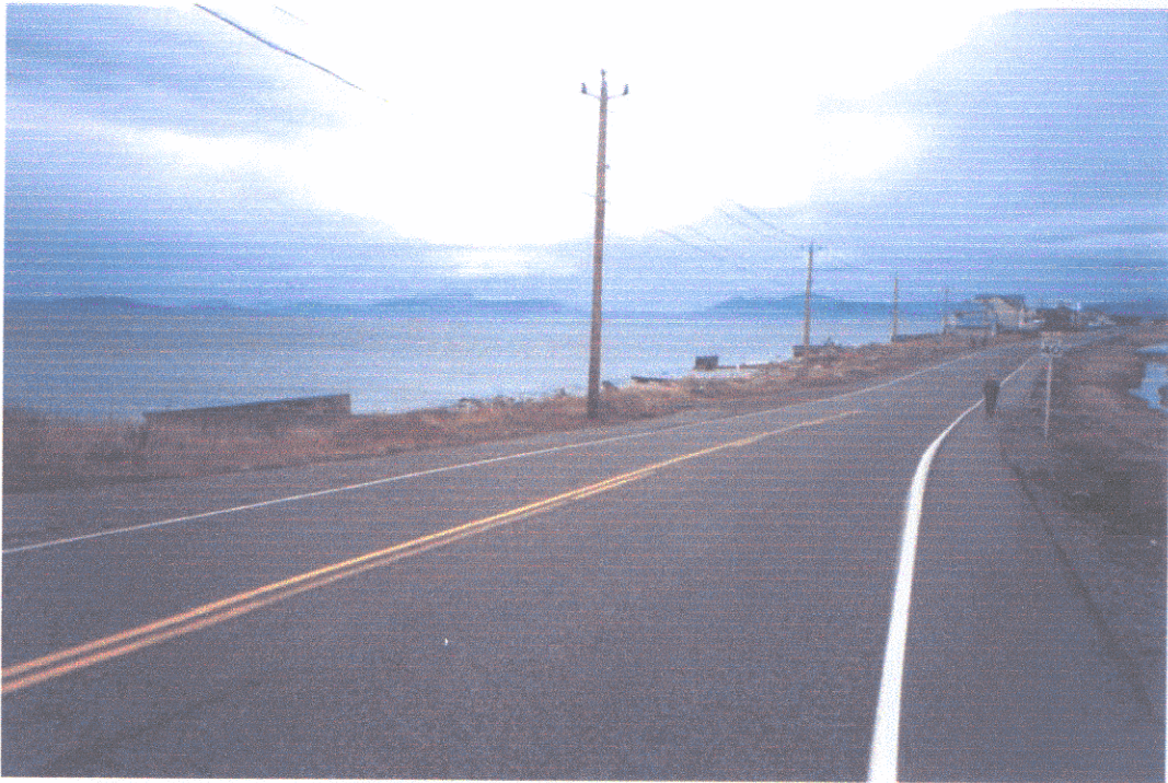
Looking north along West Beach Rd. at Strait of Juan de Fuca. Note concrete bulkheads jutting from beach.
